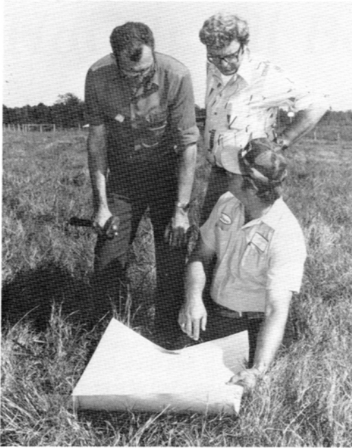
Contractor Wayne Mullenix, kneeling, goes over foundation plans with project superintendent Joe Davis (left) and Georgia Guidestones® builder Joe Fendley prior to actual work being started.
