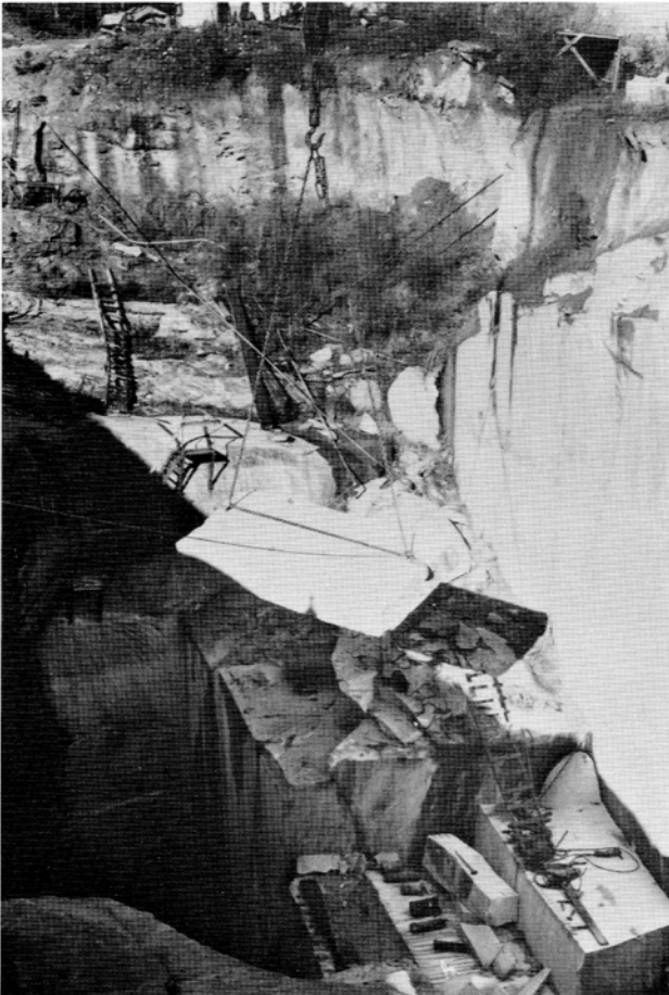
Quarrying was the most crucial phase of The Georgia Guidestones ® production because of the massive size of the granite slabs and the strain on men and equipment. It was accomplished in the more than 100-ft. depths of the "Pyramid Blue Granite" Quarry. "Our Quarry Superintendent, Jimmy Mattox, and his crew simply did a fantastic job under the circumstances," said Joe Fendley, builder of The Georgia Guidestones ® .
