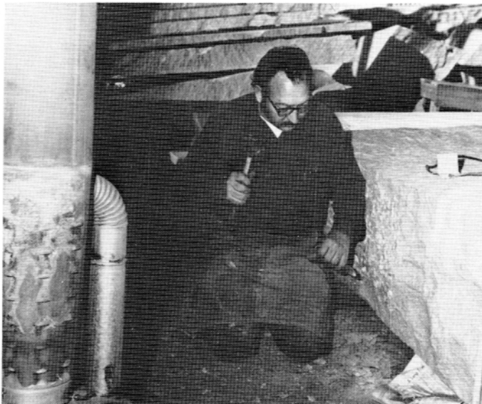
Horace Bradford, one of the two master stonecutters assigned to The Georgia Guidestones® project, is shown smoothing the sides of the center stone.
