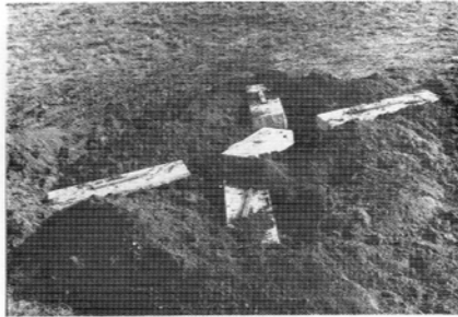
The base for The Georgia Guidestones® was set upon bed-rock and the giant "paddlewheel" is shown shortly after the concrete was poured.
