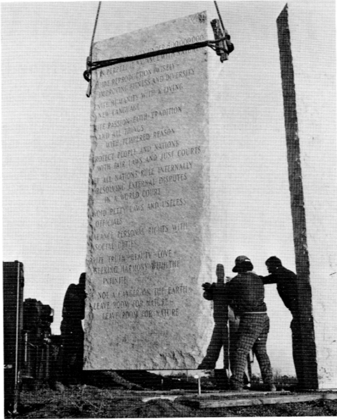
"Ever so gently!" describes how the crane and setting crew handled the stone sections and their enormous weight. As shown above, stainless steel dowell pins were placed in each of the granite bases and the upright sections were set on the pins.
